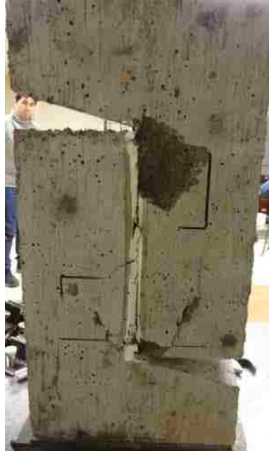
Figure 3.48 Concrete Spalling on Specimen A-SH-MO-P-2
