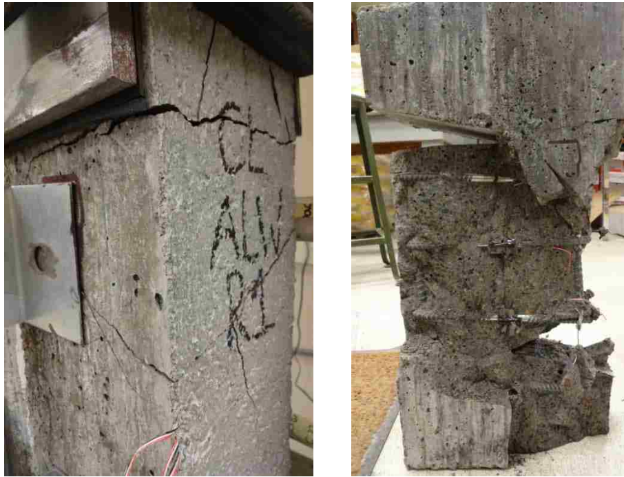
Figure 3.61 Concrete Cracking on A-CL-CJ-R-1 (left), After the Removal of All Loose Concrete (right)
